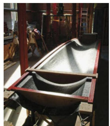
Fig. 19. Fabric mold stretched lengthwise in frame to form double curvature funicular thin-shell vault (C.A.S.T. photo)
