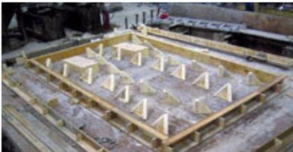
Fig. 8. Placing blockouts and interior supports prior to stretching in fabric in full scale wall panel formwork (C.A.S.T. photo)
