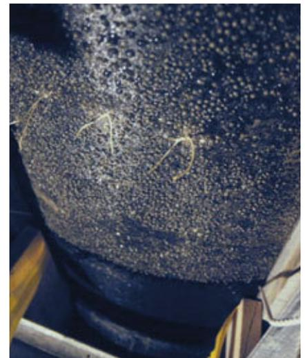
Fig. 12. Filtration of excess water and air bubbles through geotextile fabric (C.A.S.T. photo)
