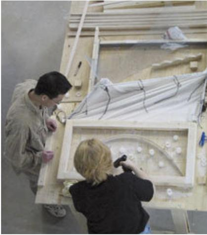
Fig. 6. Model wall panel formwork (C.A.S.T. photo)
