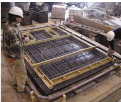
Fig. 9. Securing fabric and placing reinforcement in full scale wall panel formwork (C.A.S.T. photo)
