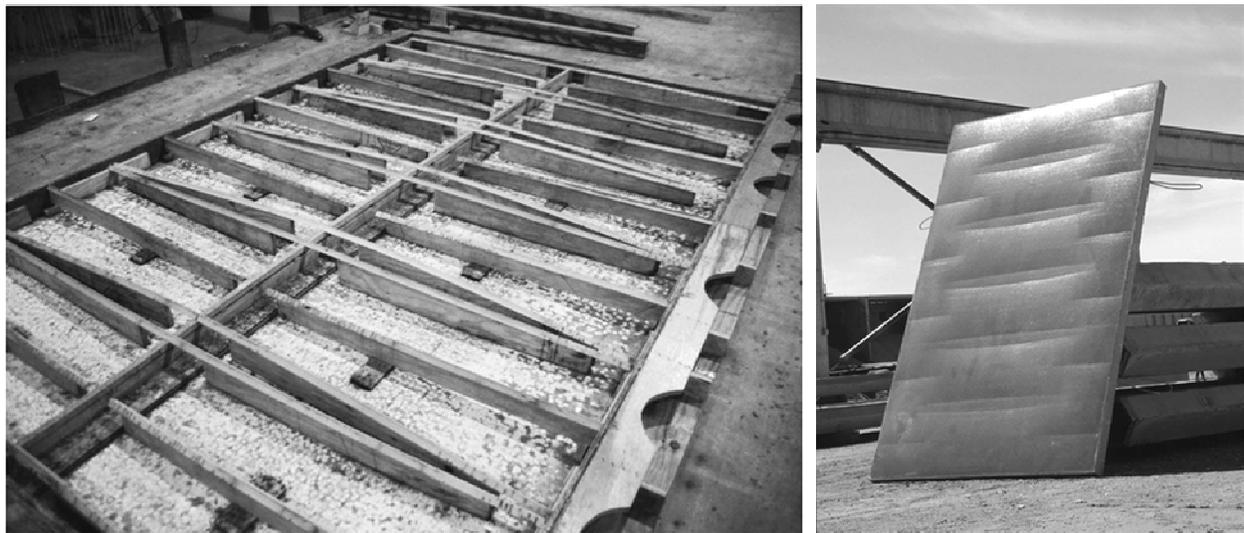
**Figure 4. Full-scale formwork and completed concrete wall panel (C.A.S.T. photos).**
