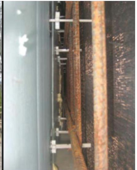
Figure 2. View of stripped formwork (left) and insulation cavity (right).
