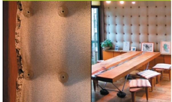
shotcrete. The inherent tensile strength of the PVC-coated or polyester fabric used for the airform allows it to be inflated to a sufficient strength to support all the applied construction materials until the concrete has cured to the point where the dome is self-supporting. Monolithic's use of fabric allowed the construction of thin-shell domes to once again be done economically.
