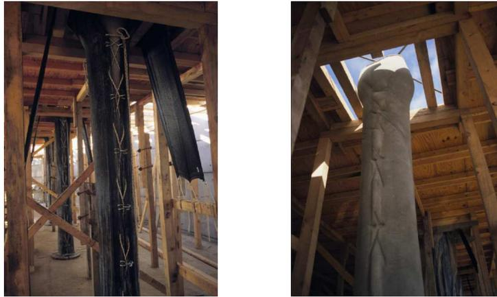
**Figure 15:** *Fabric column formwork awaiting concrete placement (left) and column after cast*
