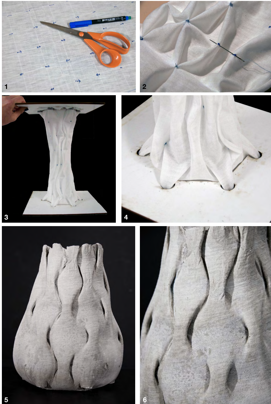
FIGURE 5.12: Column 01 (1) pattern marking, (2) sewing, (3) formwork, (4) base detail, (5) cast column and (6) surface finish detail (Source: author).
