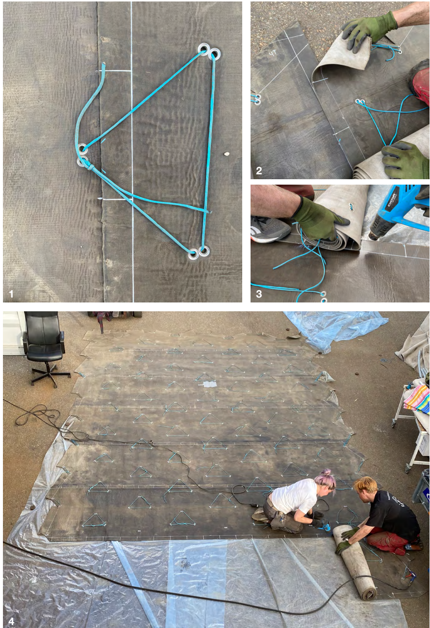
FIGURE 5.59: (1) Smock detail over a seam, (2) edge registration marks and (3,4) heat welding assembly (Source: author).
