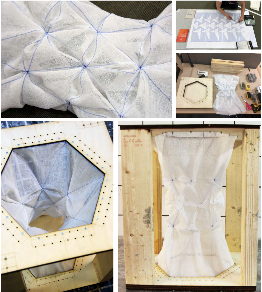
FIGURE 5.37: Column 3.2 formwork fabrication (Source: author).
