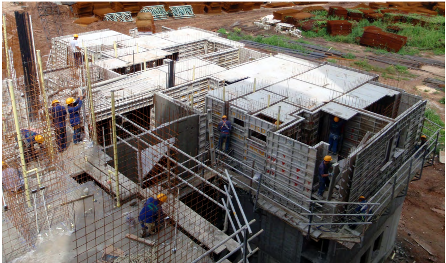
FIGURE 1.1: Traditional concrete formwork (Wikipedia Creative Commons).
