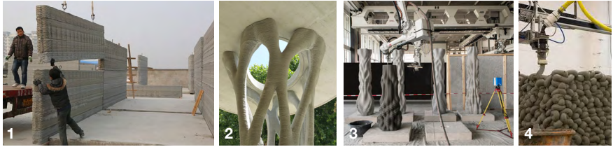
FIGURE 3.11: (1) Winsun's Concrete 3D Printed Houses (Blain, 2014). (2) XtreeE's Post (Gaudillière et al., 2019). (3) ETH's Concrete Choreography (Anton et al., 2020). (4) Kapoor's Cement Room (Kapoor et al., 2009).
