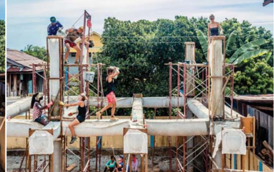
Figure 7, above left: Sewing the fabric formwork. Figure 8, above middle: Completed fabric formwork installed. Figure 9, above right: Casting upper concrete columns. Figures 10 and 11, below left and right: Completed columns at Bomnong L'or Centre.
