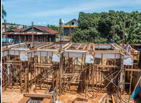
Figure 7, above left: Sewing the fabric formwork. Figure 8, above middle: Completed fabric formwork installed. Figure 9, above right: Casting upper concrete columns. Figures 10 and 11, below left and right: Completed columns at Bomnong L'or Centre.
