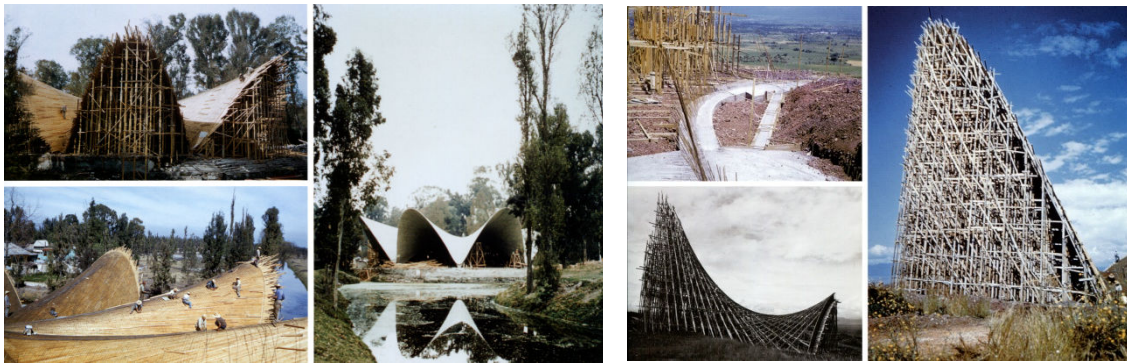
Figure 1: (left) Los Manantiales Restaurant at Xochimilco [4], and (right) Chapel Lomas de Cuernavaca [4]. Although the shape of both shells is derived from a hyperbolic paraboloid, allowing the formwork to be constructed using straight elements, it is gigantic.
