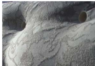
Figure 5: Detail of concrete surface showing pattern and fibres from the used upholstery fabric and exposed clamps holes.
