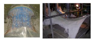
Fig. 3 Steel reinforcement before concreting
