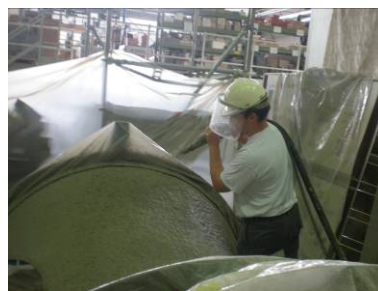
Fig. 9: Shotcrete application
