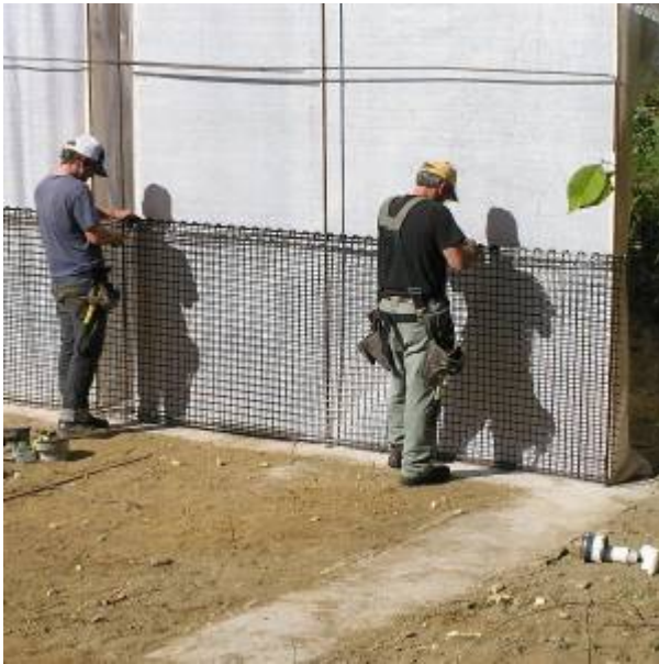
Fig. 6. Adding Carbon Fiber Grid
