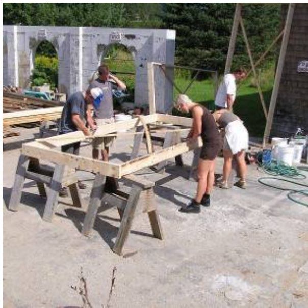
Fig. 1. Wall Form Assembly
