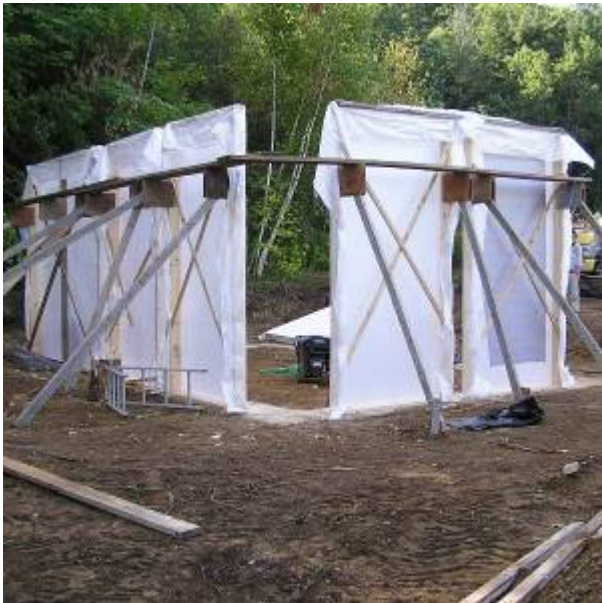
Fig. 5. Wall Form Placement
