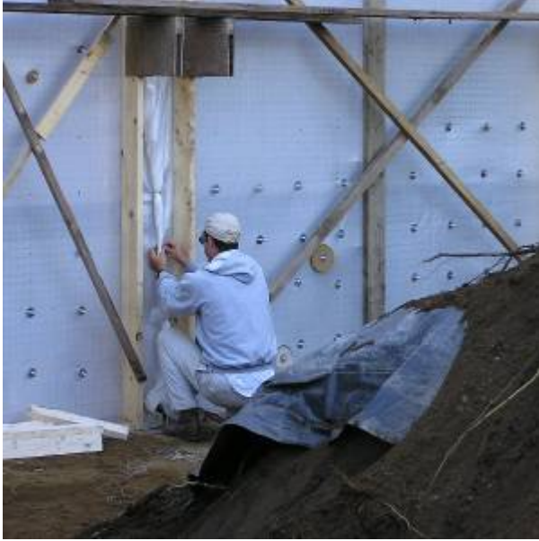
Fig. 7. Wall Form Placement
