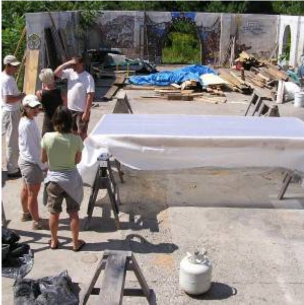
Fig. 2. Wall Form Assembly
