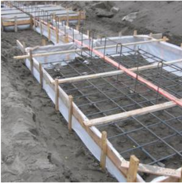
Fig. 1. Spread/Continuous Footing Application
