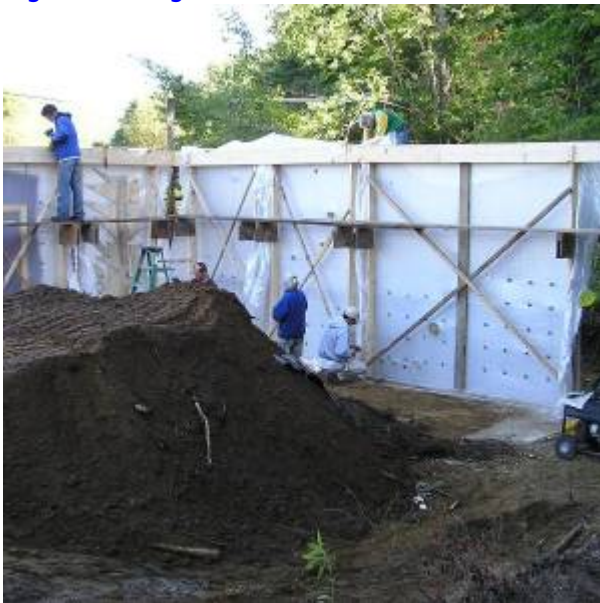
Fig. 7. Wall Form Placement
