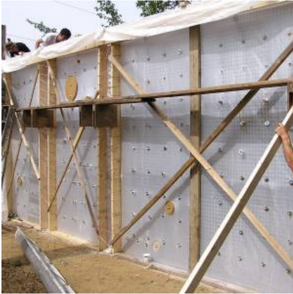
Fig. 8. Wall Form Placement
