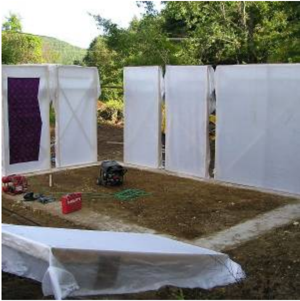
Fig. 4. Wall Form Placement
