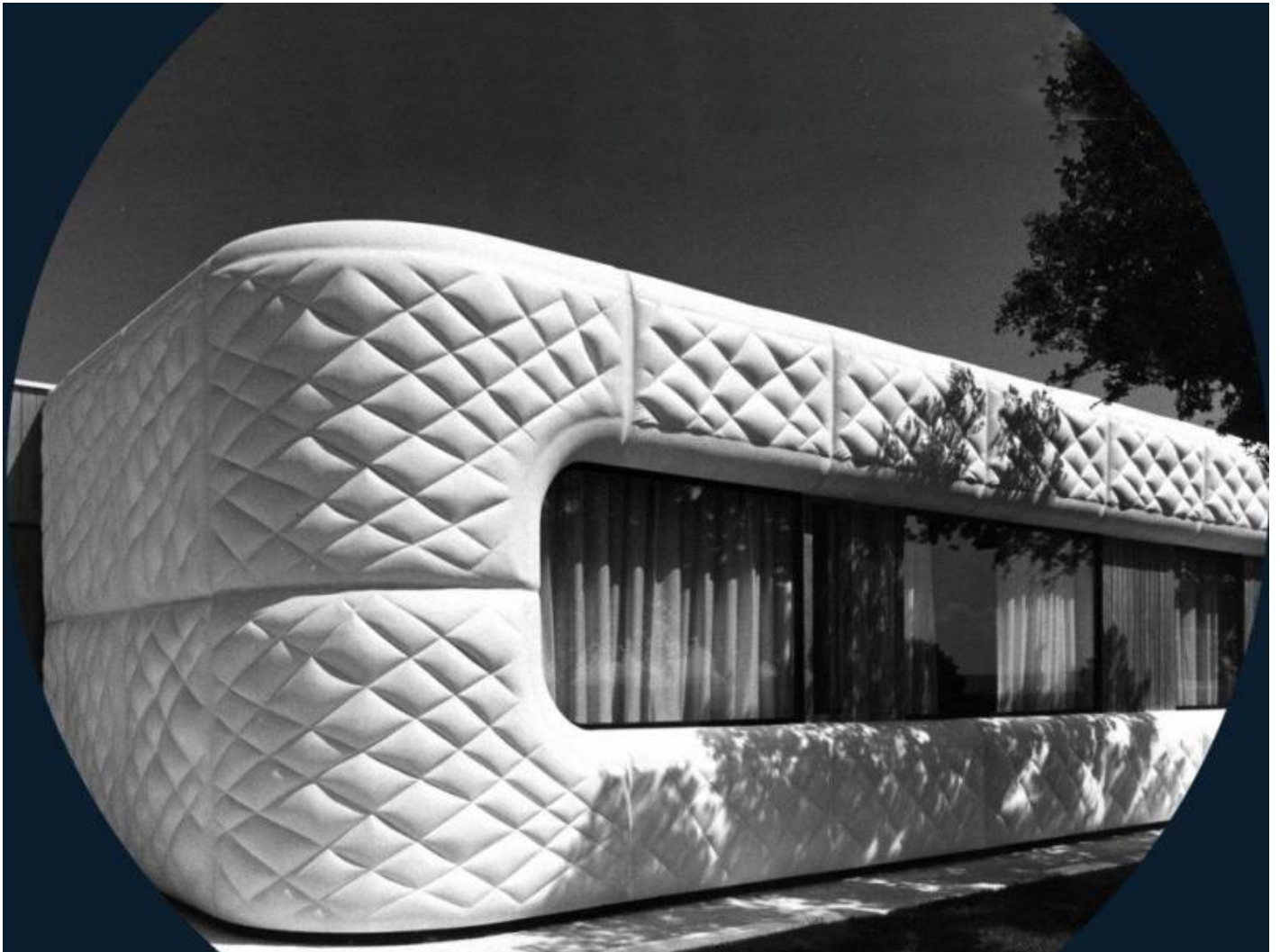
Figure 4: Prefabricated cladding for a house formed with flexible formwork and...
