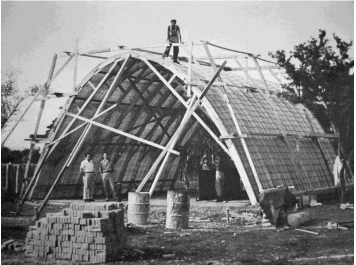
Figure 3: Vault for a rural school in Tamaulipas, Mexico, designed by Felix...
